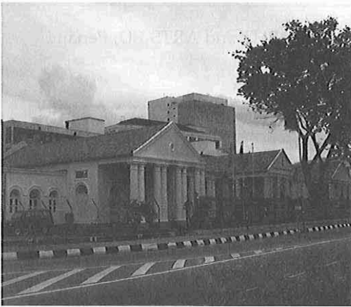
Photo 3 : State Assembly Buildings
