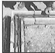
a. Stabilised rammed earth foundation and wall
