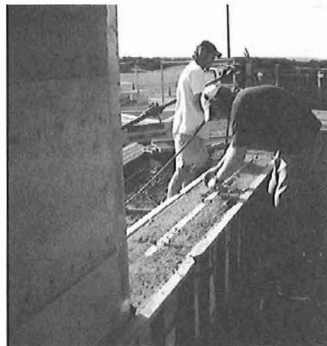
Figure 8 Rigid cavity fill insulation in composite SRE wall, photo courtesy of Earth Structures Private Ltd
